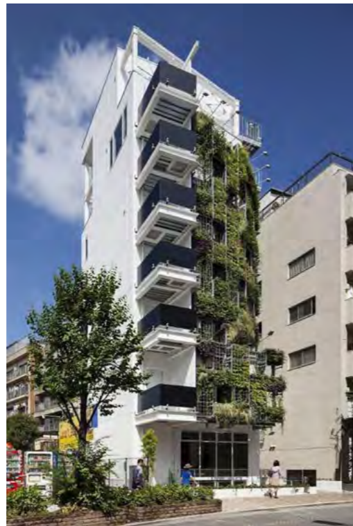
Vent Vert | Minato, Japan – Edward Suzuki Associates Inc
